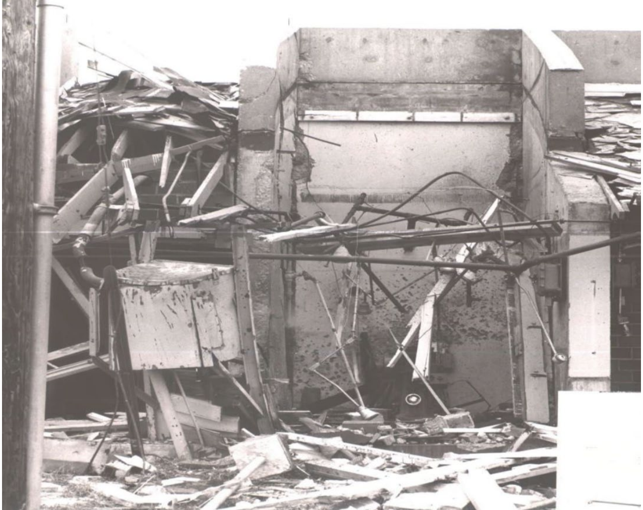
Figure 8 – In this photo of the donor cubicle, deformations of the side walls are particularly apparent.
