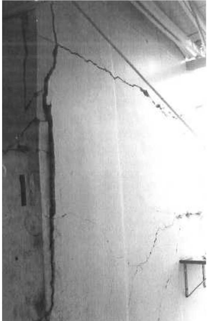
Figures 6 – The photo on the left depicts the diagonal tension and direct shear cracks in a donor cubicle's wall. The photo on the right shows a severe direct shear crack along the vertical, side/rear wall joint.
