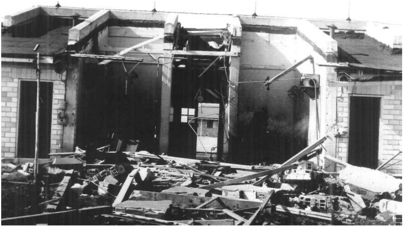
Figure 2 – Damages sustained by donor and acceptor cubicles when the dividing walls which separate them do not extend to the exterior wall.
