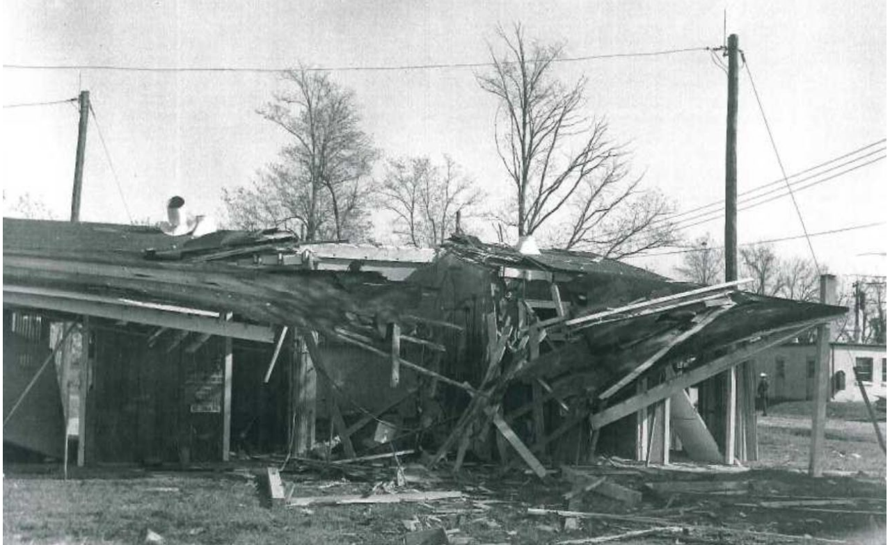
Figure 7 – Enhanced damage and debris hazards when donor and acceptor cubicles share a common roof.
