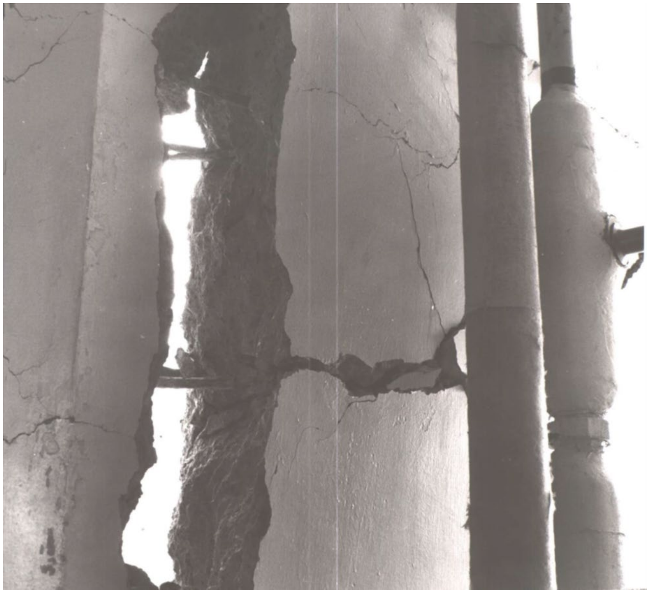
Figure 9 – Severe direct shear cracking along a side/rear wall joint in the donor cubicle
