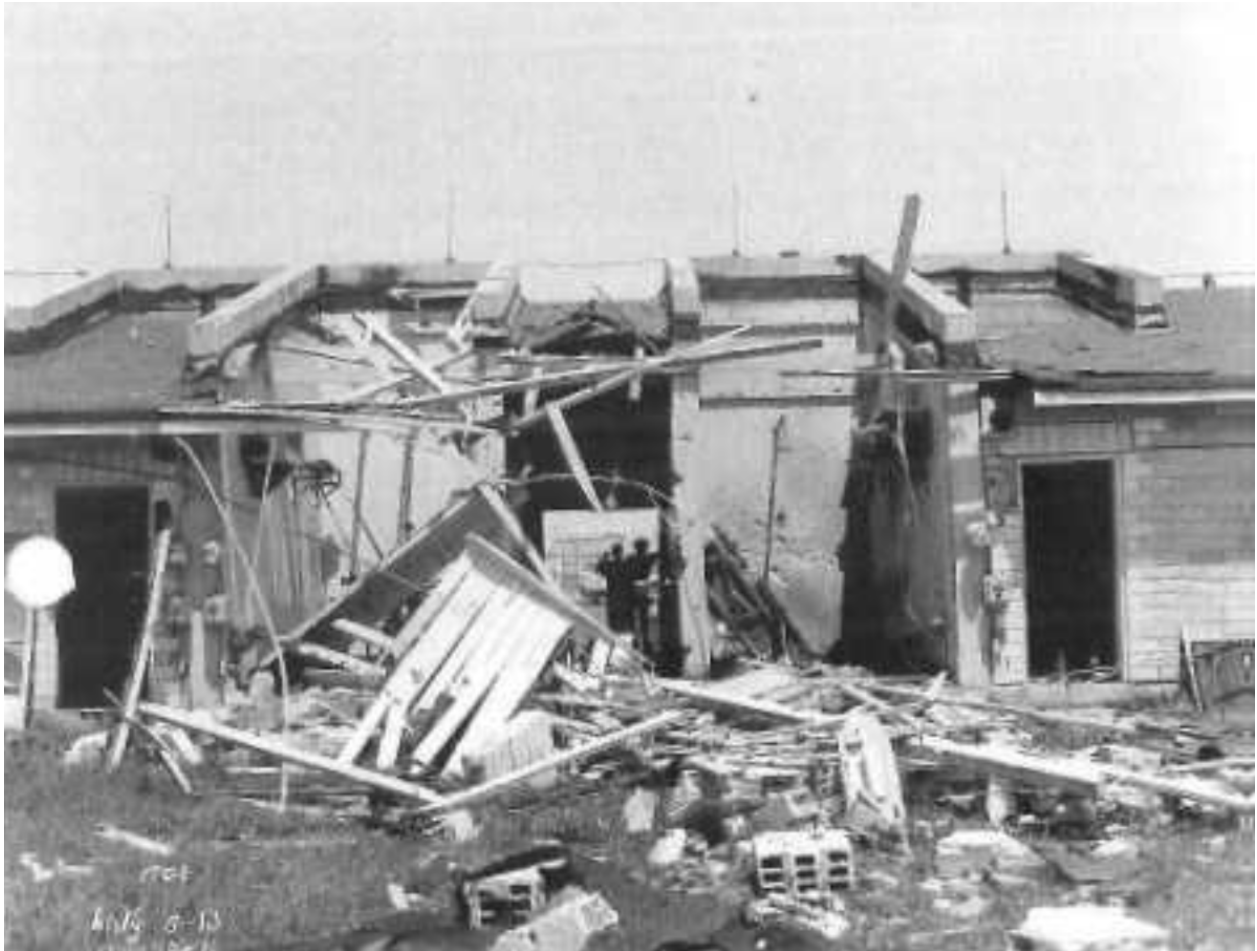
Figure 5 – Similar to accident 1, the 12-inch SDWs separating the donor and acceptor cubicles did not extend to the exterior wall, increasing the damage to the acceptor cubicle.
