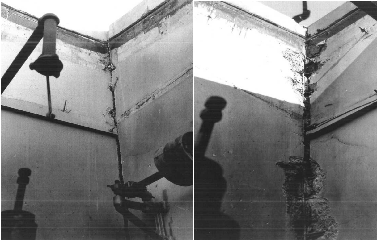
Figure 3 – Direct shear cracks along the vertical side/rear wall joints of the donor cubicle.
