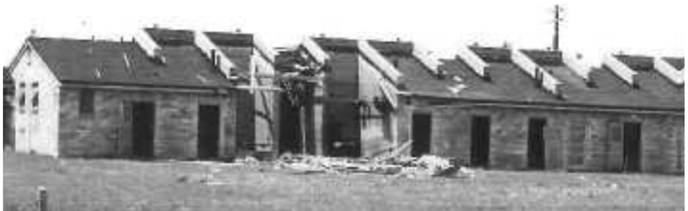
Figure 1 – Damages sustained by a typical, WWII-era explosives operating building in an accidental detonation.
